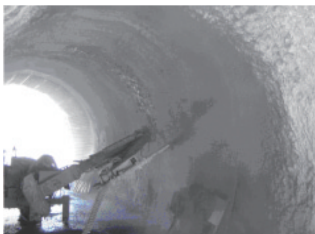
Fig.2-6 State of shotcreting in the test tunnel
