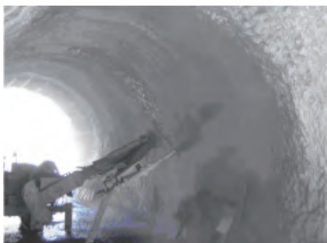
Fig.2-6 State of shotcreting in the test tunnel
