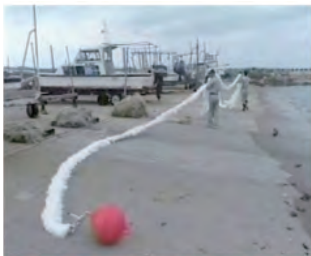
Fig.4-12 Preparing braided adsorbent for mooring on sea bottom
