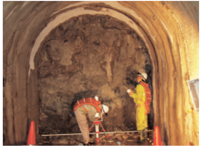
Geological inspection of a sub stage horizontal tunnel at the depth of 200m
