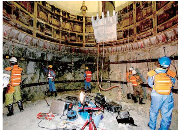
Geological mapping at the bottom of main shaft
