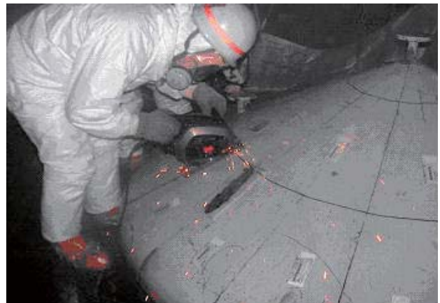
Decommissioning status of the Refinement and Conversion facility
