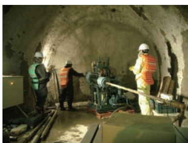
(c) Borehole ① drilling situation
