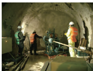
(c) Borehole ① drilling situation
