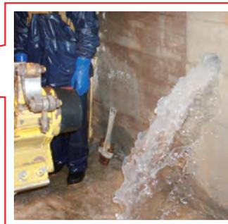
**Fig.14-25 Water inflow from injection-hole of the pre-excavation grouting**
