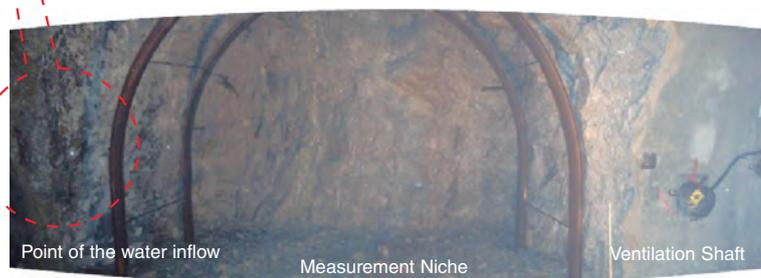
**Fig.14-26 Tunnel and wall of GL-200m Measurement Niche off Ventilation Shaft**
