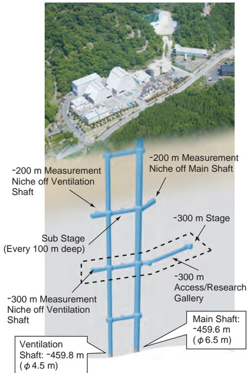
**Fig.14-25 Layout of the Mizunami Underground Research Laboratory**
