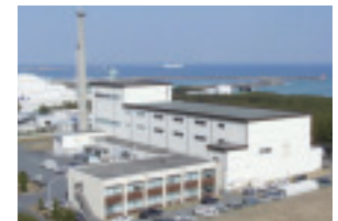
Reactor Fuel Examination Facility
