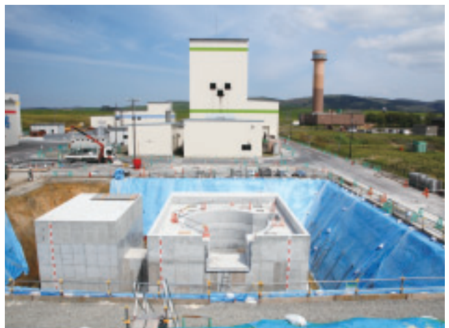
West Access Shaft (photo 2011.6.1)
