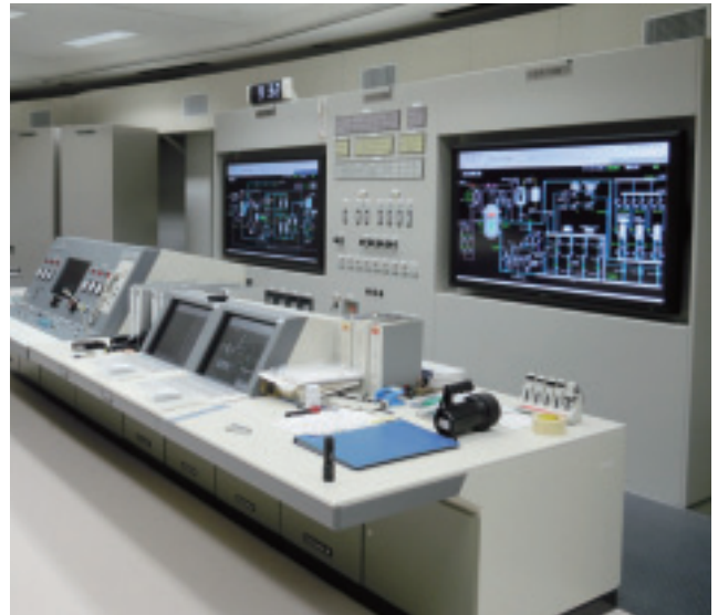
Renewed instrumentation and control system in JMTR control room
