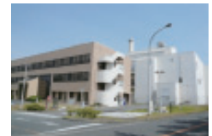
Nuclear Fuel Cycle Safety Engineering Research Facility (NUCEF)
