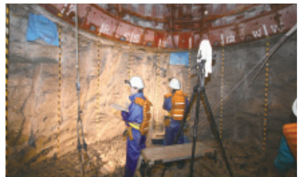
Fig.12-28 Geological mapping underway in the Ventilation Shaft
