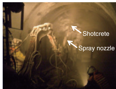
Fig.2-23 Spraying HFSC shotcrete in the drift
