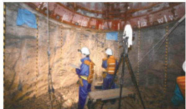
**Fig.12-28 Geological mapping underway in the Ventilation Shaft**
