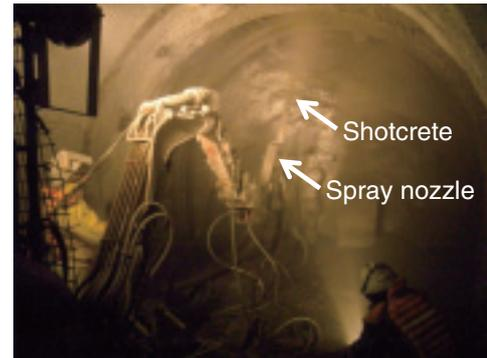
**Fig.2-23 Spraying HFSC shotcrete in the drift**
