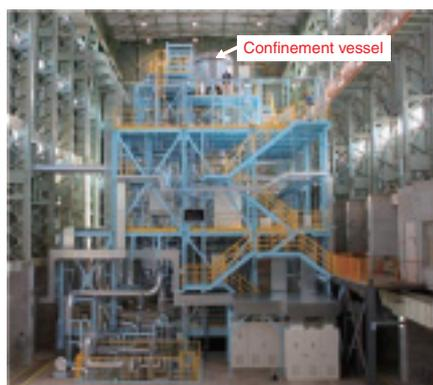
**Fig.3-27 IFMIF/EVEDA Li Test Loop (ELTL) after completion of construction**
