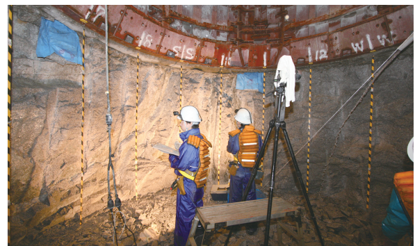
Fig.12-28 Geological mapping underway in the Ventilation Shaft
