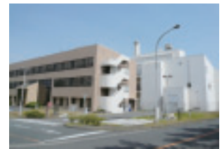
Nuclear Fuel Cycle Safety Engineering Research Facility (NUCEF)
