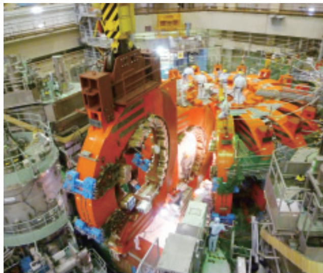
Disassembly operation of TF coils in JT-60 (December 2011)
