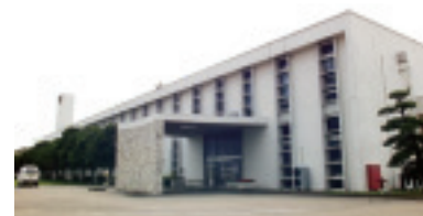
Plutonium Fuel Development Facility
