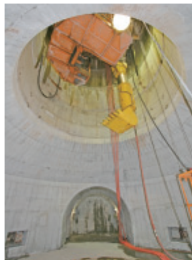
View of the intersection of the Main Shaft and the horizontal tunnel at the GL -500 m stage
