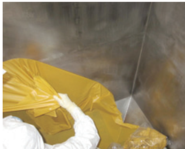
This photograph shows the state of decontamination of a tank obtained using a commercially available decontamination reagent. The commercially available decontamination reagent, which became a film, is peeled off in the figure.
