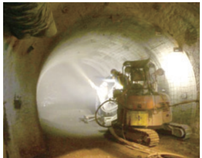
Spraying test of low-alkaline cement in the 250 m Gallery off the west shaft
