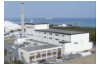
Reactor Fuel Examination Facility
