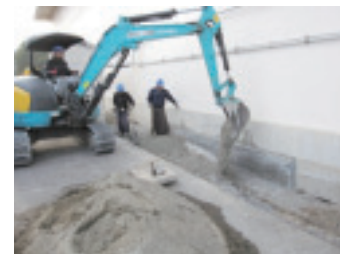
Fig.13-8 Recycling of the concrete debris
