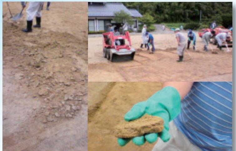
Decontamination of soil by using poly-ion complex in Oguni, Ryozen, Date-city, Fukushima
