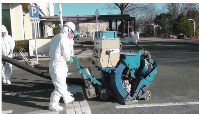
Fig.1-15 Shot blasting (the Okuma town government office area)
