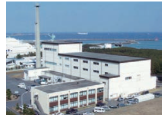
Reactor Fuel Examination Facility
