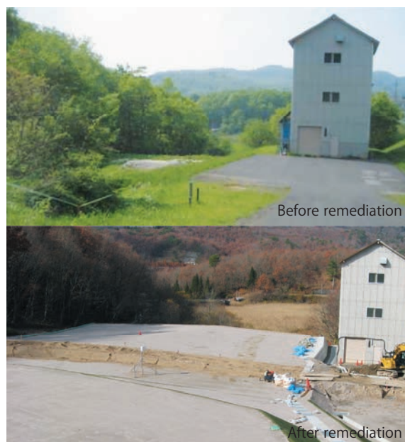
Upstream part of the Yotsugi Mill Tailings Pond
