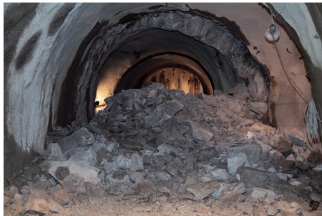
Breaking through at part of the GL -500 m Sub Stage (July 30, 2012)
