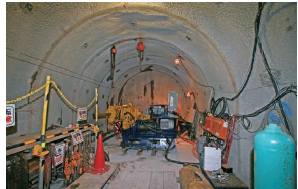
Fig.13-23 Borehole investigation site
