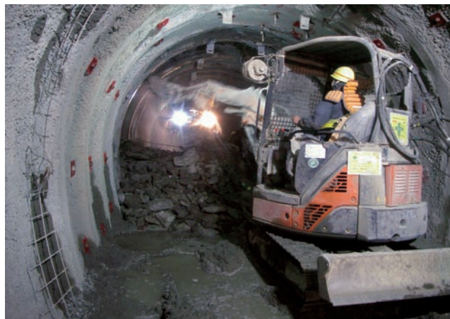
Penetration of 350 m research gallery between the ventilation and east shafts
