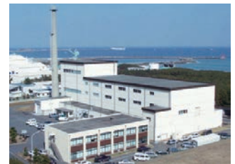
Reactor Fuel Examination Facility
