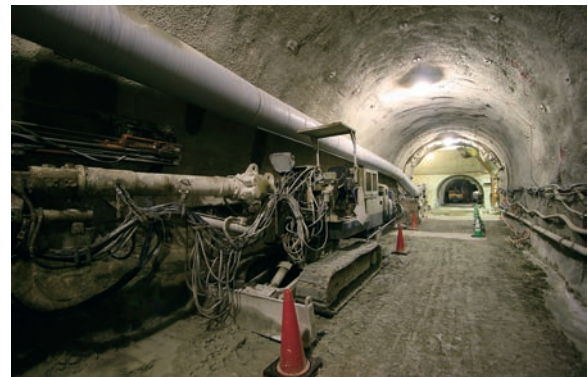
Fig.13-22 -500 m Access/Research Gallery-North
