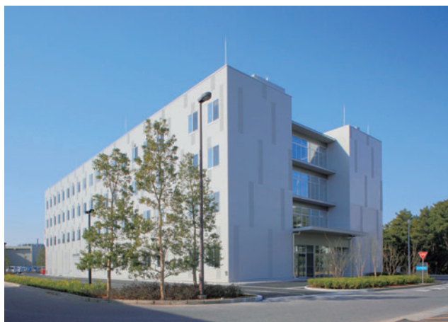
Fig.5-1 Photo of the J-PARC Research Building
