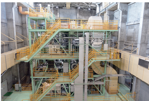
Fig.7-2 Plant-dynamics test loop
